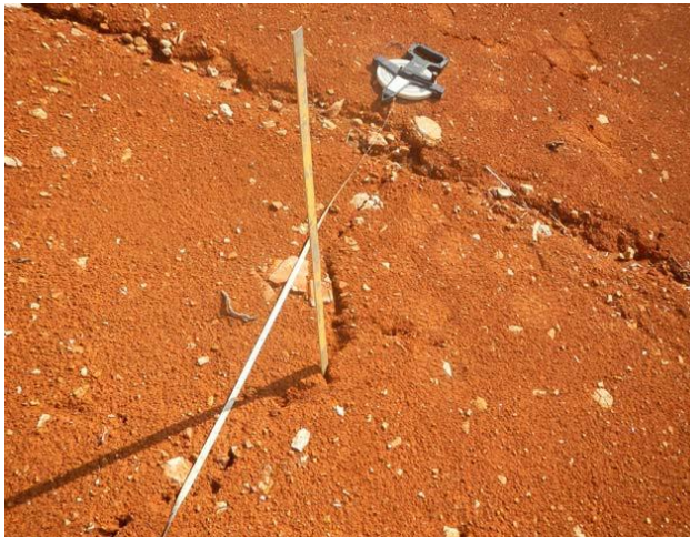
Figure 7. The clay liner shown here is the sole confining entity separating the hog waste in the lagoons from the underlying Boone Formation. This photo, taken after construction of the liner, indicates that it has numerous chert fragments up to fist size within the clay, that it has desiccation cracks, and that erosion rills have eroded some of the thickness. These features reduce its ability to confine. It was required to be 30 cm thick, but the owners of the CAFO increased that to 45 cm. (Photo courtesy of Tony Morris, ADEQ).
