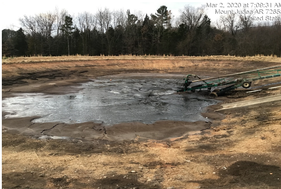
Photograph 20: Pond 1 with nearly all liquid waste removed.
