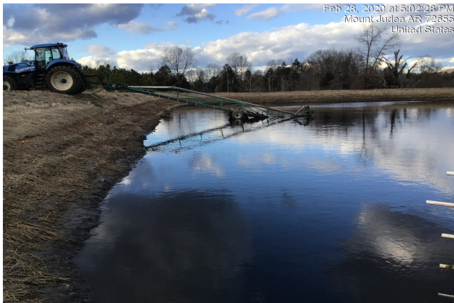
Photograph 18: Removal of liquid waste from Pond 2 continued.
