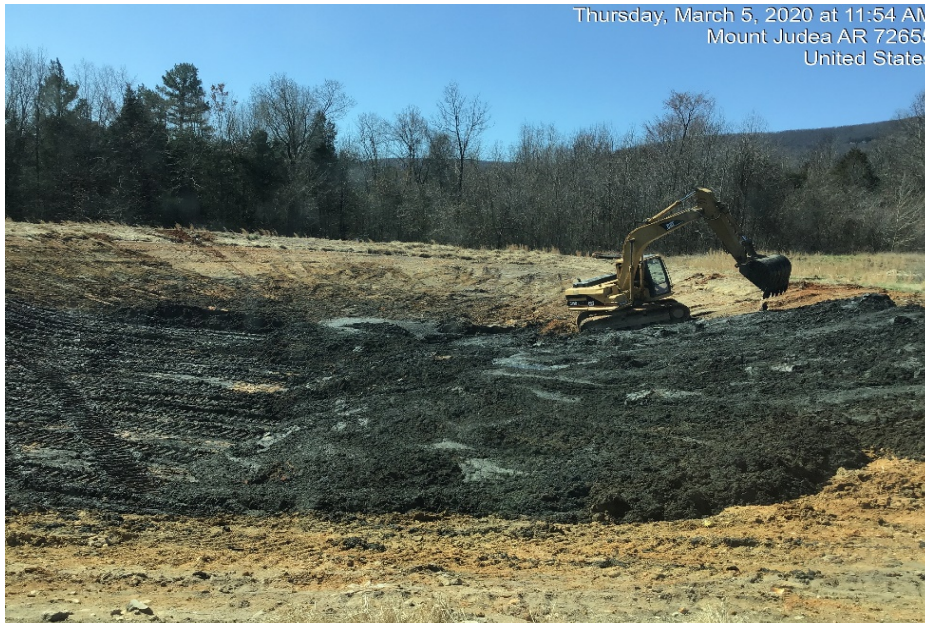
Photograph 26: Solid waste is removed from from Pond 1.
