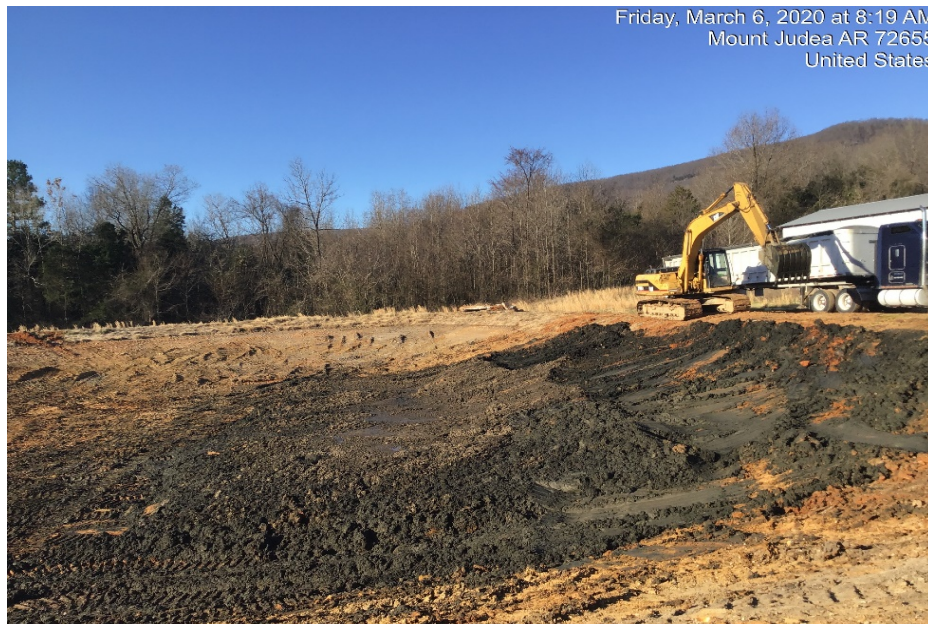
Photograph 27: Removal of solid waste from Pond 1 continued.
