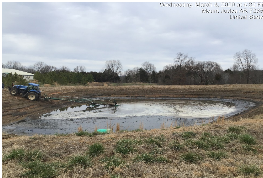
Photograph 24: Removal of liquid waste from Pond 2 continued.
