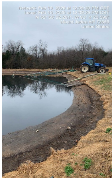
Photograph 11: Removal of liquid waste from Pond 1 continued.
