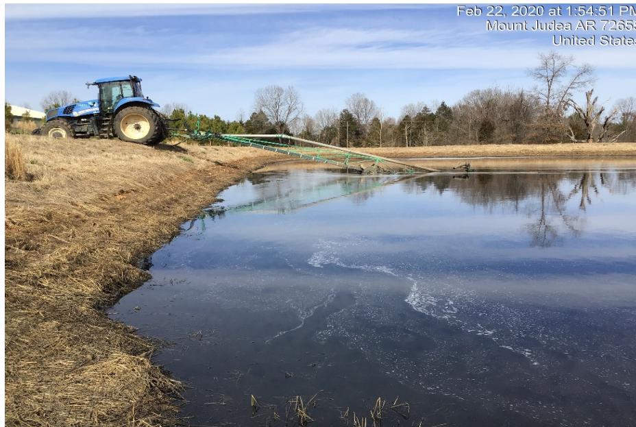
Photograph 16: Removal of liquid waste from Pond 2 continued.
