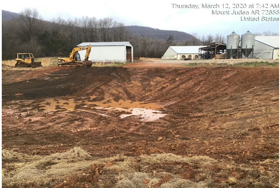
Photograph 29: Removal of solid waste from Pond 1 continued.
