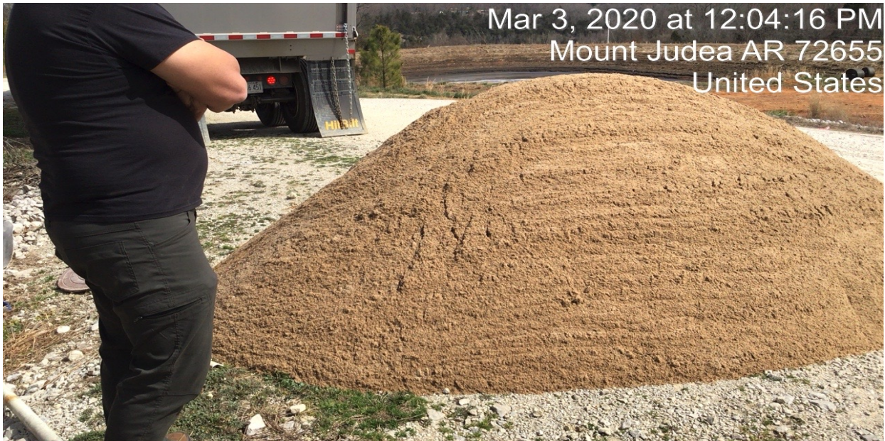
Photograph 22: Manhole was filled with sand.
