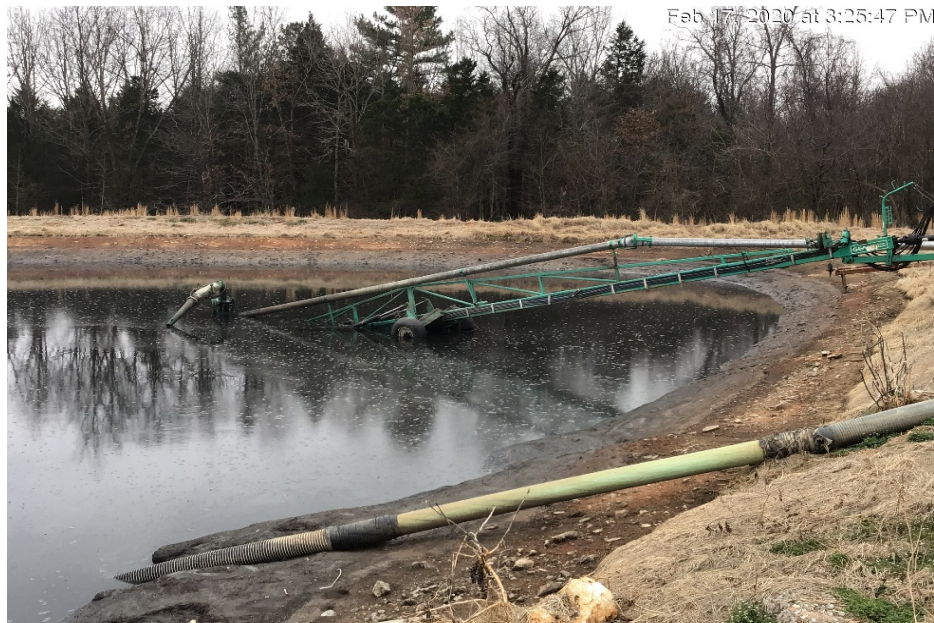
Photograph 12: Pumping of liquid waste from Pond 1 continued.
