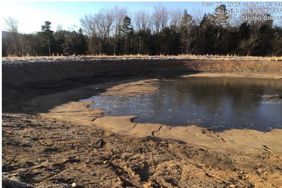
Photograph 17: Pond 1 nearly all liquid waste removed, solid waste remaining. Rainfall resulted in more liquid waste to be removed.
