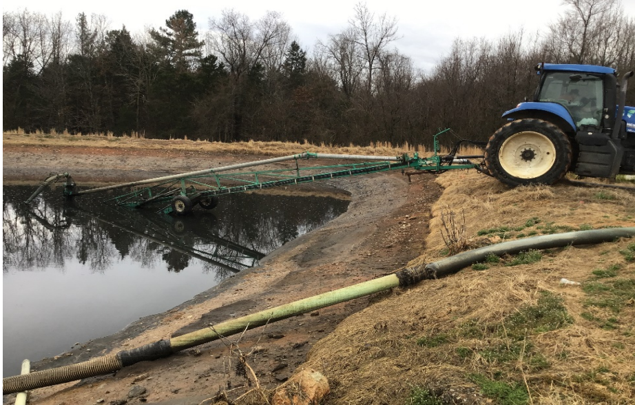
Photograph 13: Pumping of liquid waste from Pond 1 continued.
