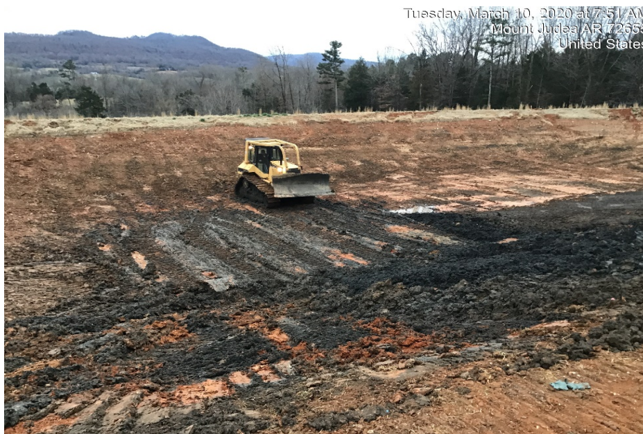
Photograph 28: Removal of solid waste from Pond 1 continued.
