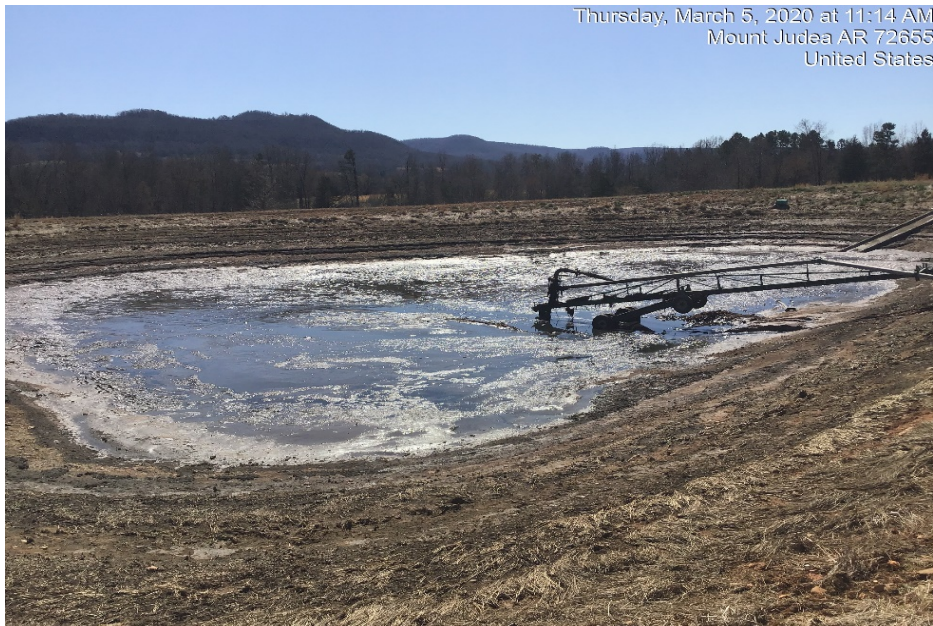
Photograph 25: Removal of liquid waste from Pond 2 continued.
