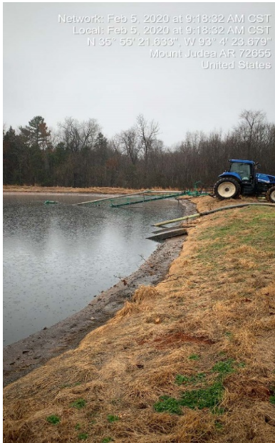
Photograph 7: Removal of liquid waste from Pond 1 continued.
