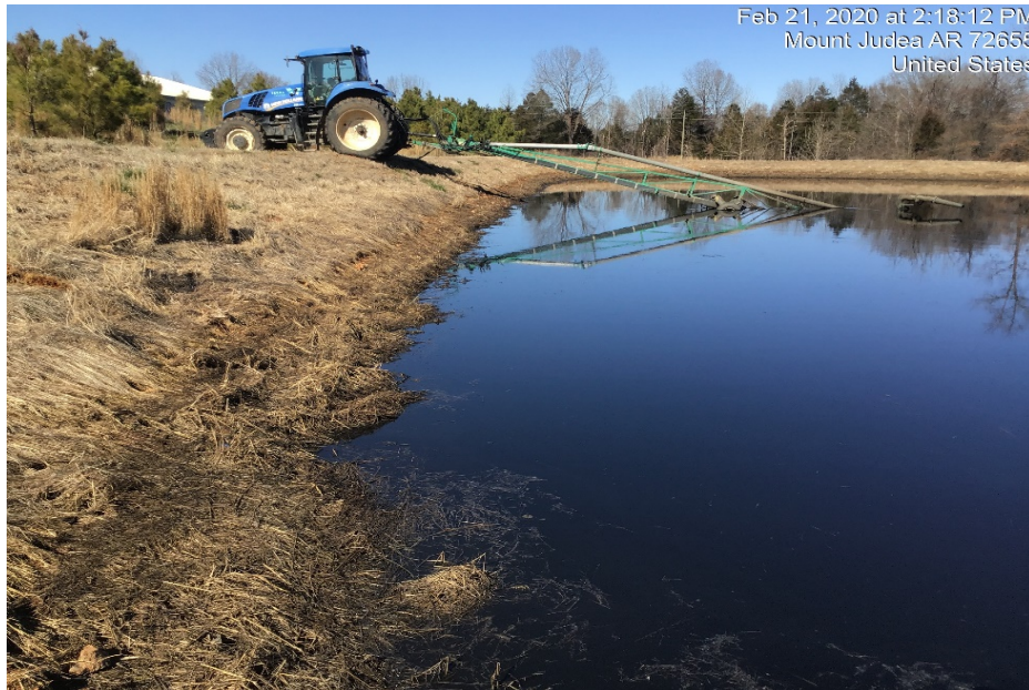
Photograph 15: Removal of liquid waste from Pond 2 started.
