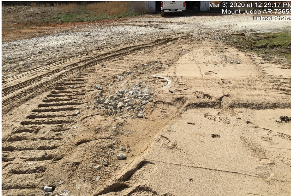
Photograph 23: Manhole filled with sand.
