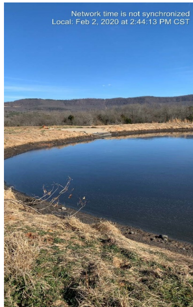
Photograph 4: Water level of Pond 1 after one (1) day of pumping liquid waste out.
