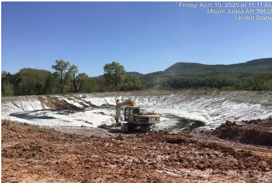
Photograph 48: Lime was added to solid waste in Pond 2 to help solidify solid waste.
