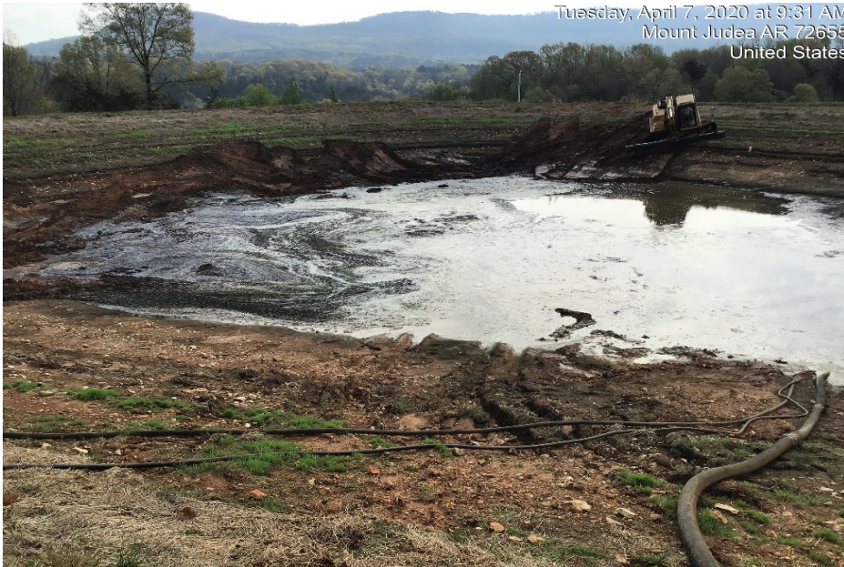
Photograph 44: Pond 2, with most liquid waste removed. Mainly solid waste remained.
