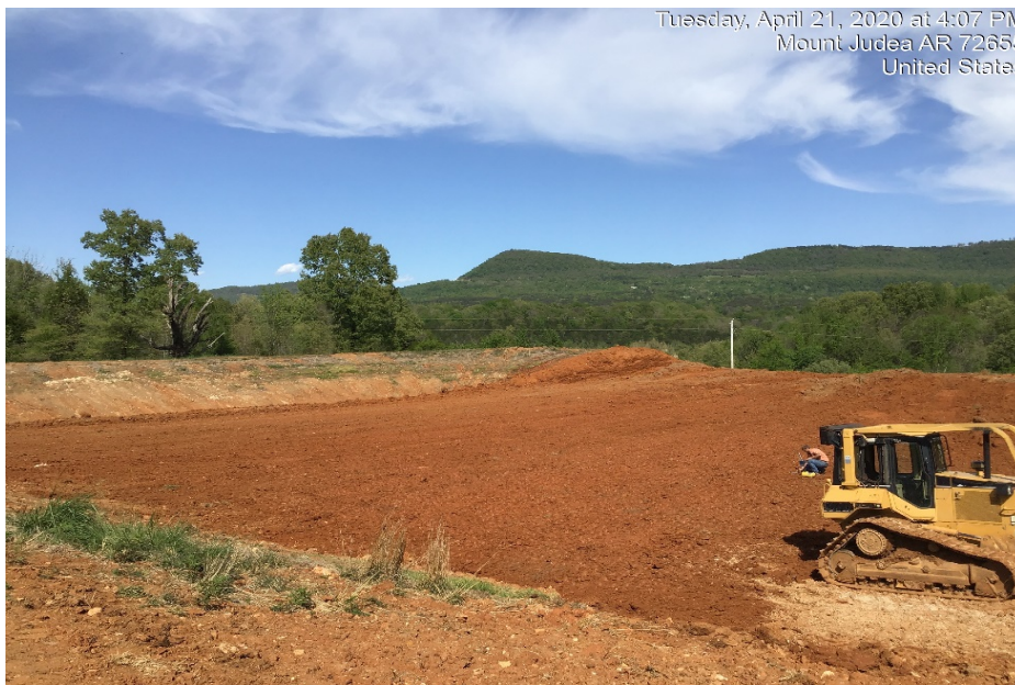
Photograph 54: Material being placed in compacted lifts over Pond 2 continued.
