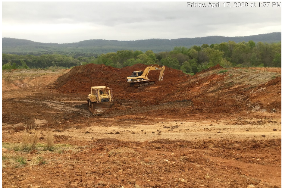
Photograph 51: All solid waste has been removed from Pond 2 and levee was breached to ensure rainfall resulted in no additional liquid waste.
