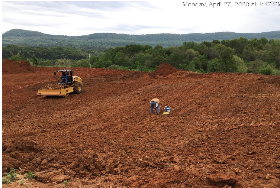
Photograph 55: Soil density testing was conducted on every lift placed.
