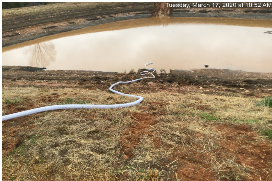
Photograph 31: Removal of liquid waste from Pond 2 continued. Additional rainfall resulted in additional liquid waste to be removed.
