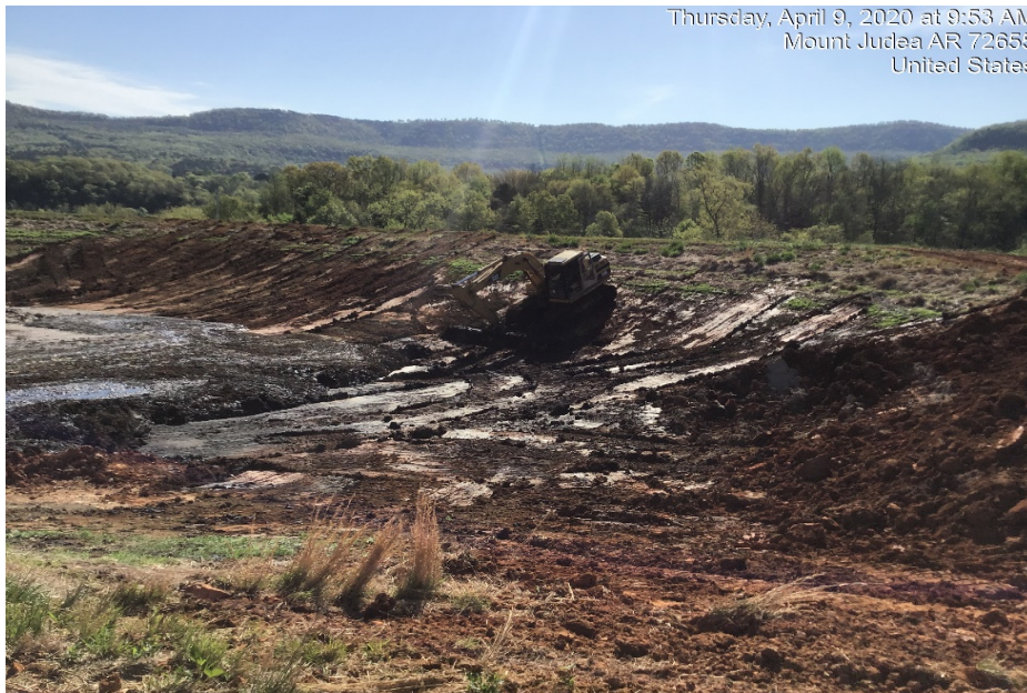
Photograph 47: Solid waste was removed from Pond 2.
