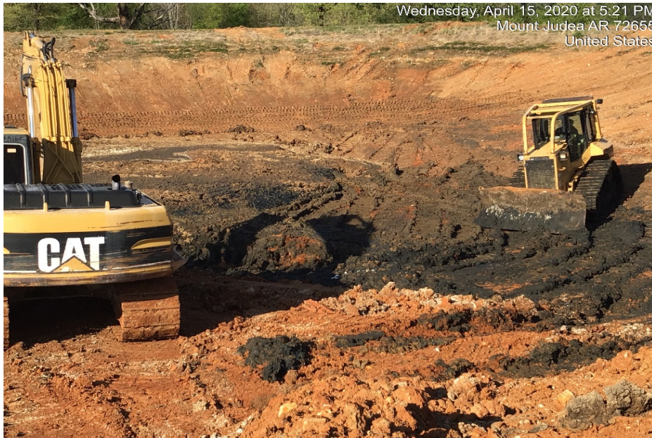
Photograph 50: Solid waste was removed from Pond 2.
