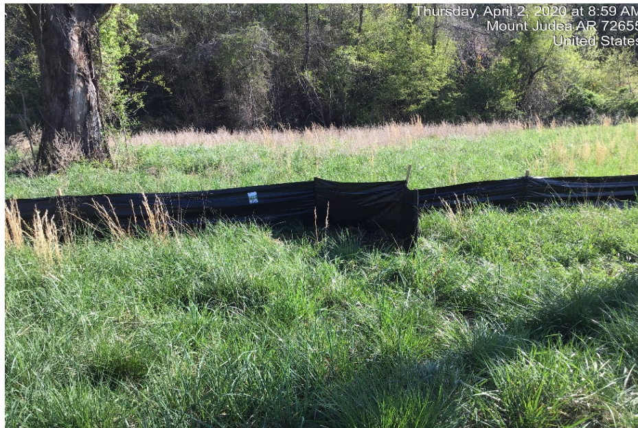
Photograph 41: Slit fence surrounding site was placed.
