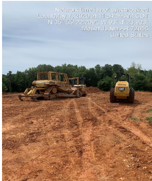
Photograph 58: Material being placed in compacted lifts over Ponds 1 & 2 continued.
