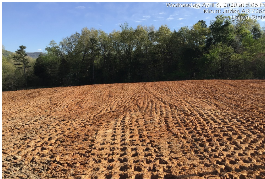
Photograph 46: Material has been placed and compacted over Pond 1.
