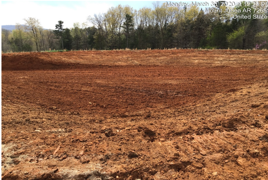
Photograph 38: Pond 1 with all liquid and solid waste removed.
