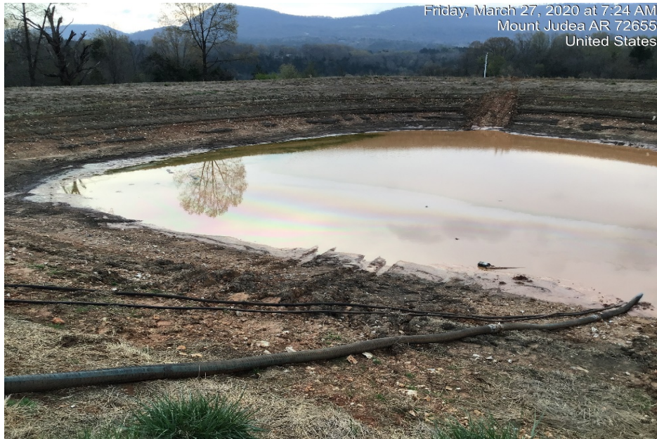
Photograph 35: Removal of liquid waste from Pond 2 continued.
