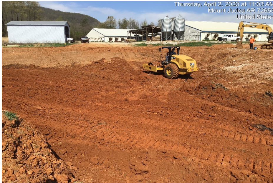
Photograph 43: Material was placed in lifts over Pond 1.
