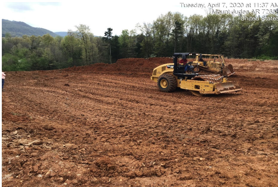
Photograph 45: A lift of material being compacted over the old Pond 1.
