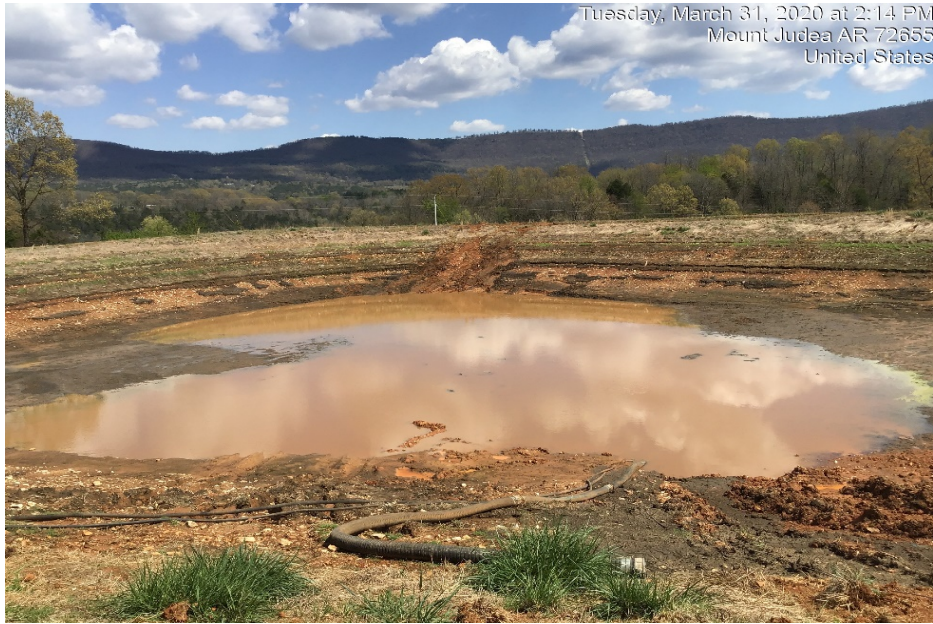
Photograph 39: Additional rainfall resulted in additional liquid waste to be removed from Pond 2.
