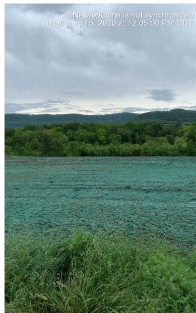
Photograph 60: Installation of bonded fiber matrix.
