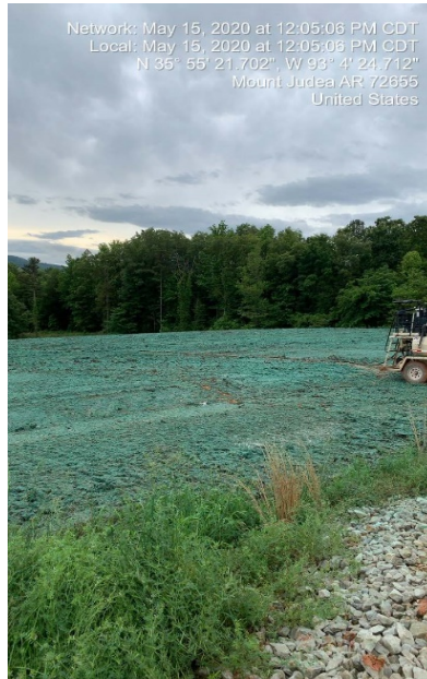
Photograph 61: Installation of bonded fiber matrix.
