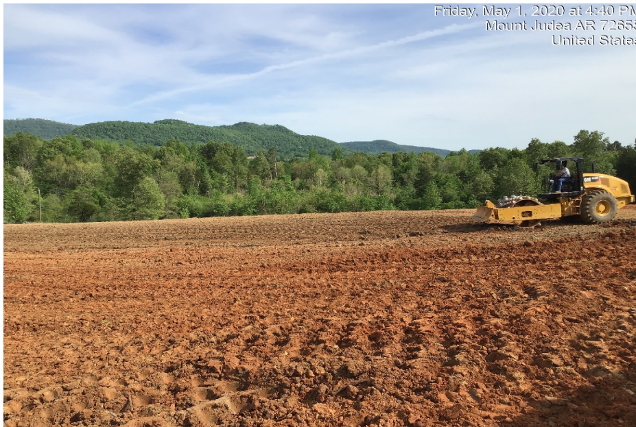
Photograph 56: Material being placed in compacted lifts over Pond 2 continued.
