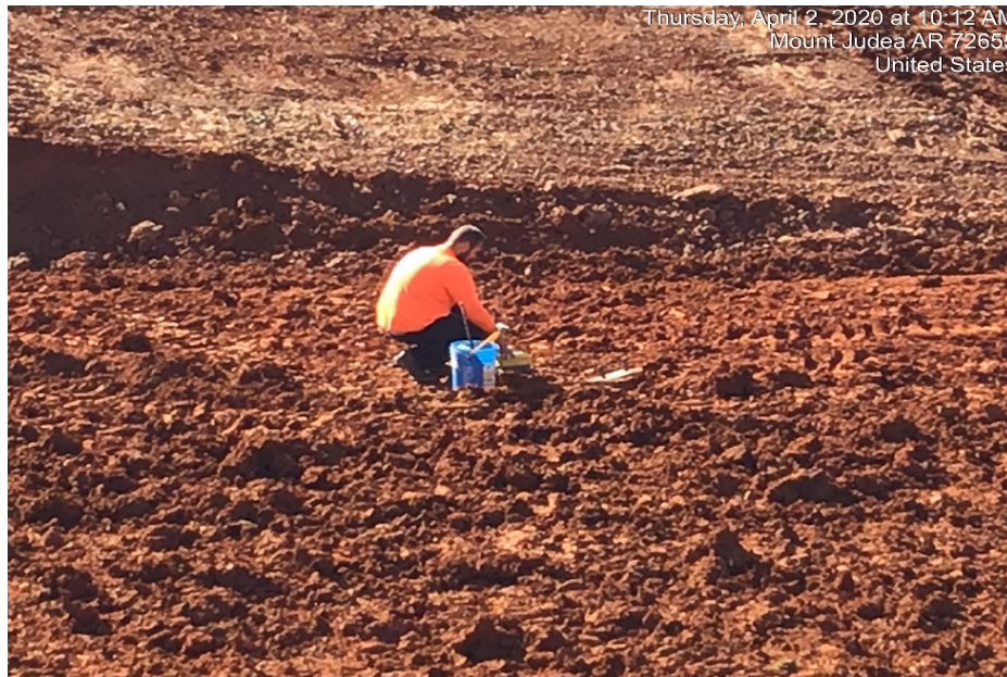
Photograph 42: Soil density testing was required for each lift of material placed.
