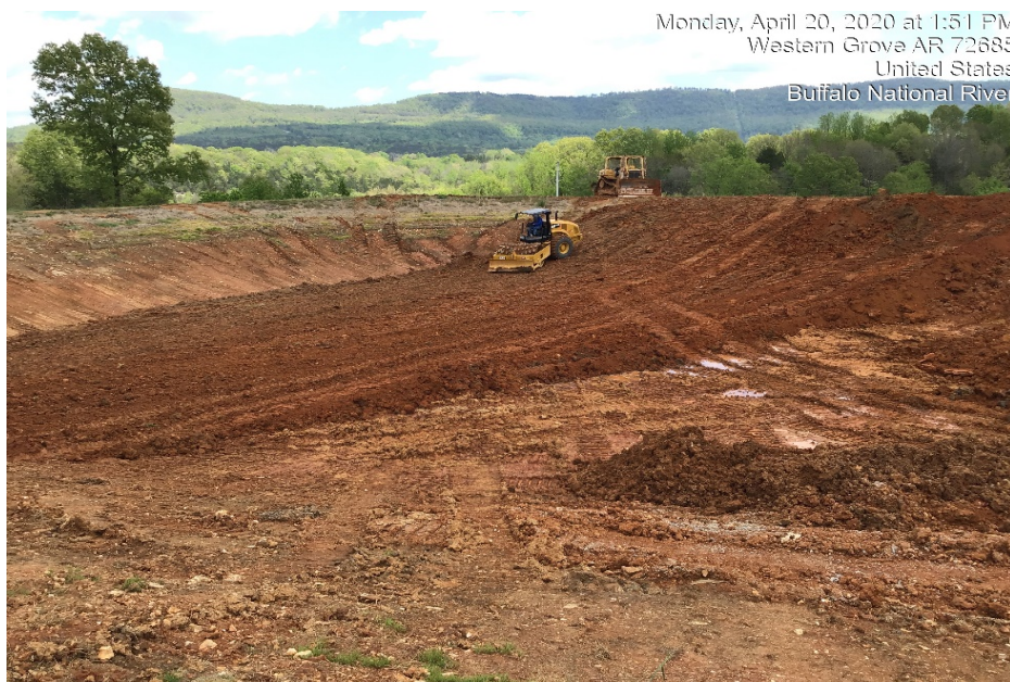
Photograph 53: Material was placed in compacted lifts over Pond 2.
