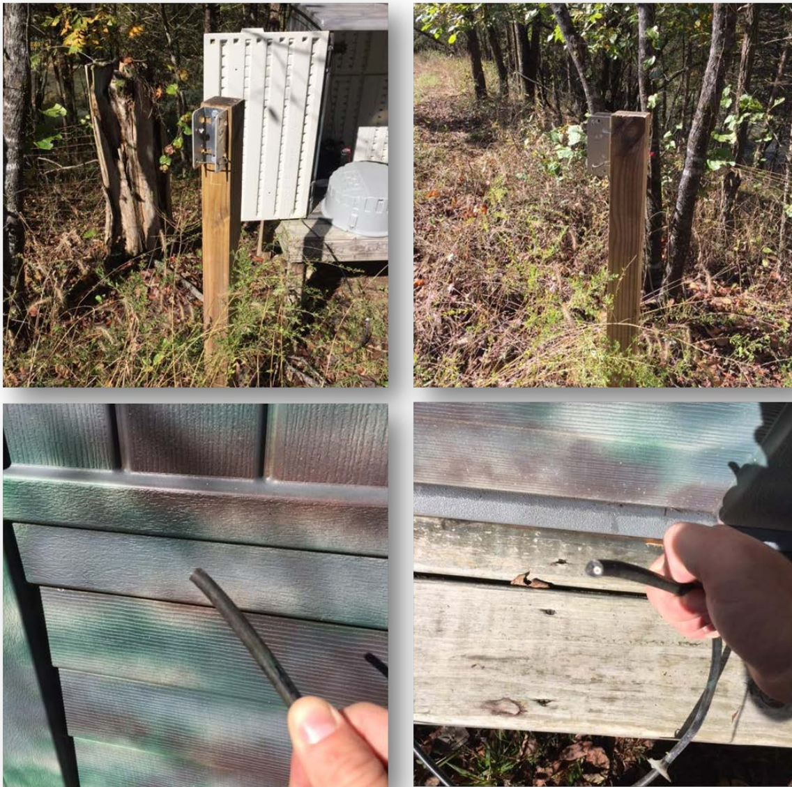
Figure 3. Missing solar panel and cut connecting cable at site BC7, downstream of the C&H Farm on Big Creek.
