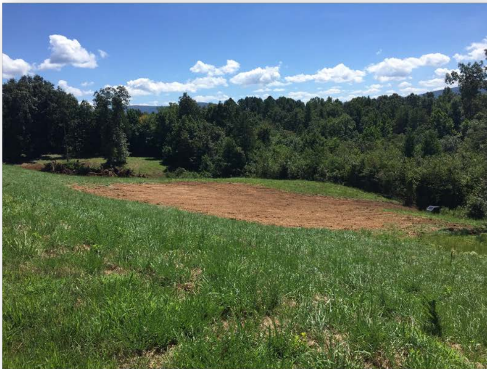
Figure 2. Reshaped land above trench 1 and 2 at the C&H Farm.
