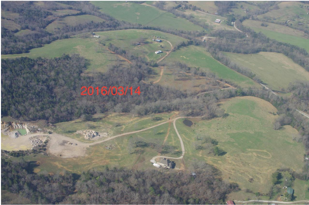
FIGURE 6 AERIAL VIEW OF FIELDS 2 AND 3 SHOWING COW TRAILS AND OTHER EVIDENCE OF ERODIBLE CONDITIONS.
