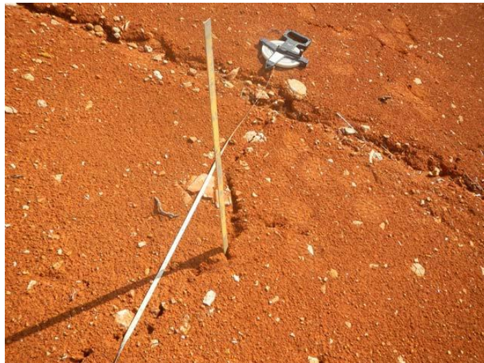
FIGURE 3 LINER CRACKS (FROM INSPECTION REPORT BY ADEQ, TONY MORRIS 7/23/2013)
