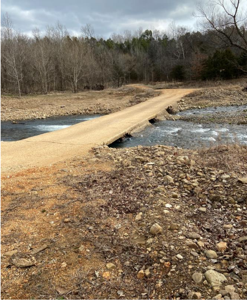
Figure 8. Newton county road 264 crossing Cave Creek near Bass.
