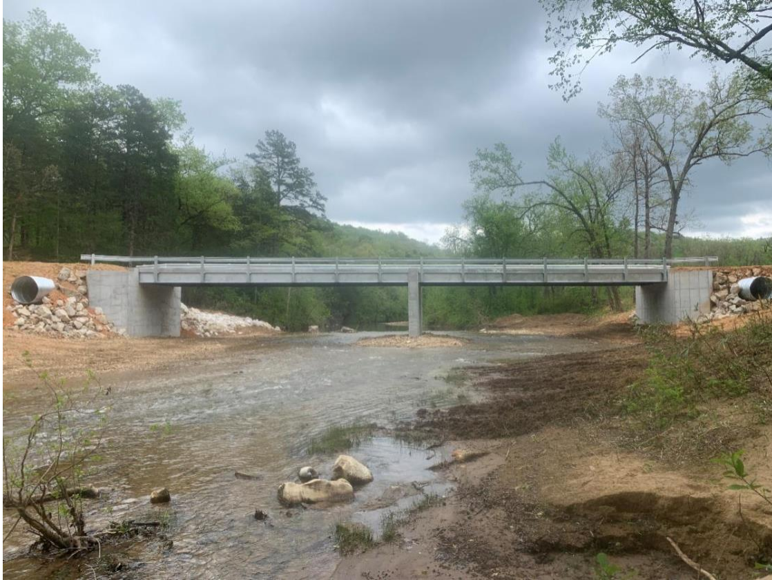
Figure 7. Completed new crossing for Newton County road 252.
