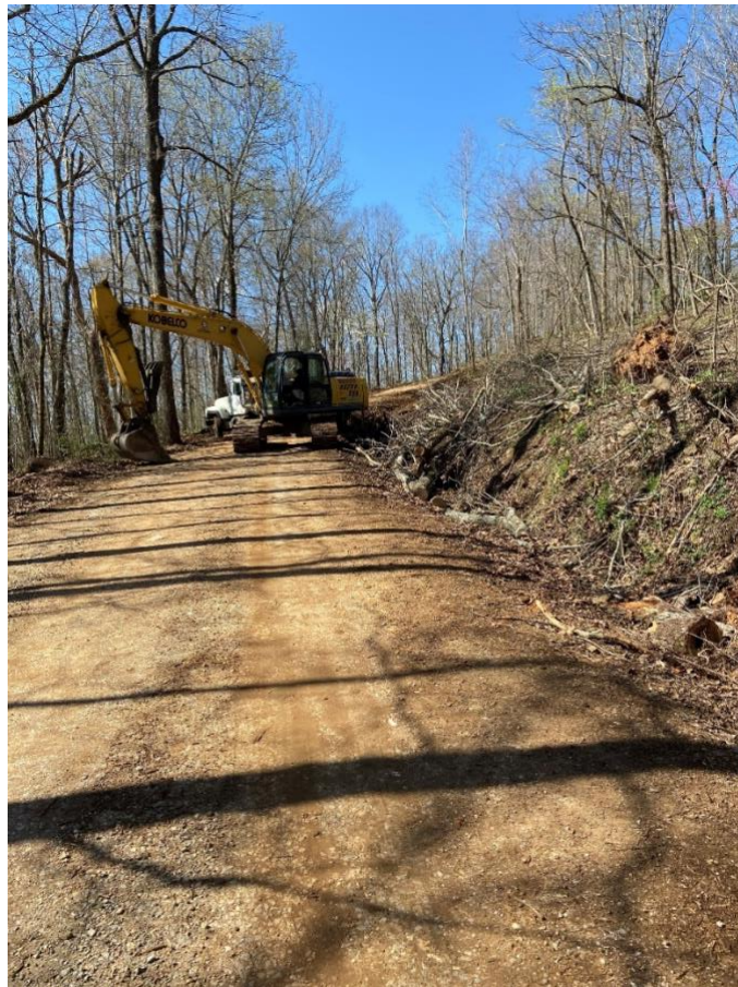
Figure 1. Cave Mountain project site in early April 2021 during debris removal.
