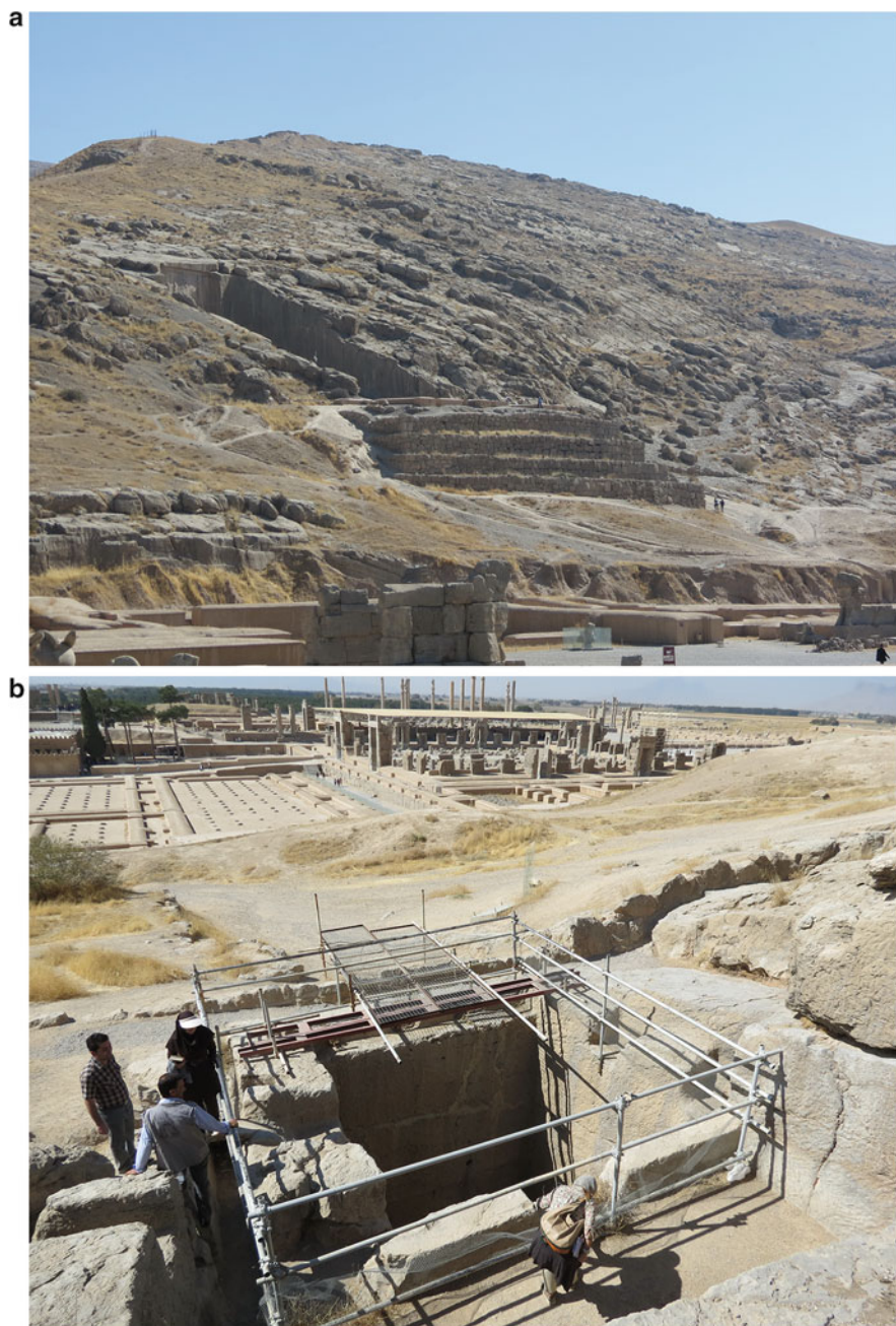
Fig. 9 (a) Sarvak limestone Fm. (Upper Cretaceous) at the edge of Persepolis, (b) “The Stone Well” quadratic shape shaft was excavated to supply the city with potable water
