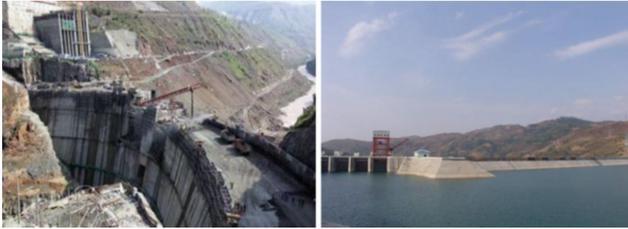
Fig. 7 The Trunk Dam construction (left) and the reservoir (right) on the Karst areas
