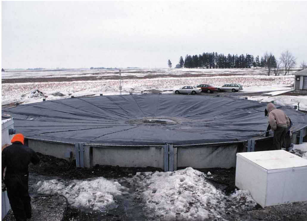
Figure 7.6. Covered manure tank generating methane in Iowa.
