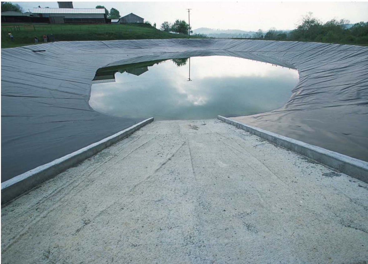
Figure 5.5. A new lagoon with a synthetic geotextile liner to prevent seepage into groundwater.
